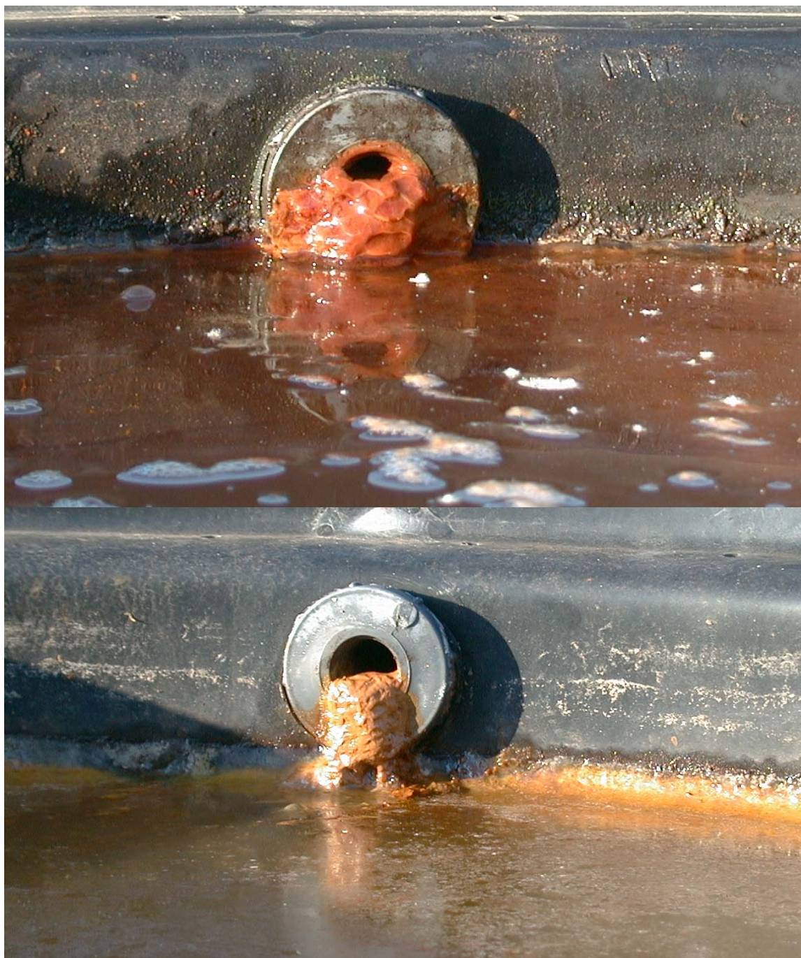
Figure 5. Photographs of the tank influent orifice showing iron oxyhydroxide crust precipitated at pH \sim 2.4. These low pH iron oxyhydroxides crusts may have played a significant role in the sorption and retention of arsenic from the influent ARD.
